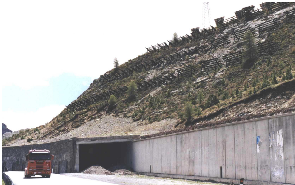
Figure 6. An example of both snow supporting structures and an avalanche shed or gallery for roadway avalanche hazard defense.
